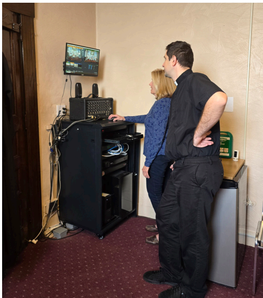
Arleen Jama and Father Vitalii Stashkevych check broadcasting equipment at SS. Peter and Paul in Braddock, Pa.
